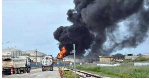
SEVERELY HIT. An industrial building and a fuel tanker at Israel's oil refineries in Haifa were hit by debris from an intercepted Iranian missile REUTERS
